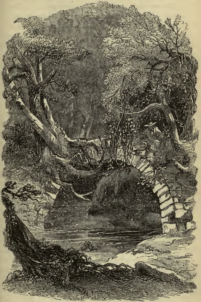
ANCIENT BRIDGE AT OLD PANAMA.
